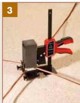
Close the mould cover. Following steps including ignition and clean up jobs are similar to the case of specific moulds.
