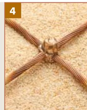
Carefully remove the cavity sealer to check the result. Be aware: the system is at an extremely high temperature.
