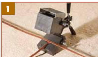
Place the conductors in the mould and close the handle clamps to avoid material leakages during the reaction.
