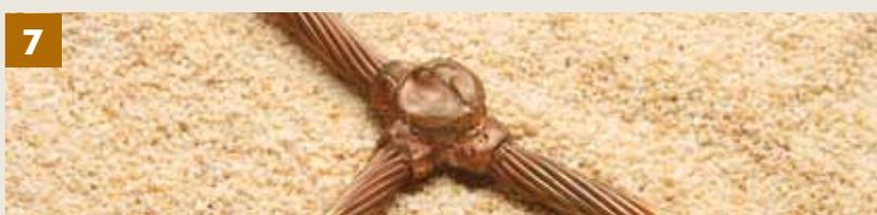
Once open, clean the slag stick to the mould with the relevant clearing brush. Then the mould will be ready to be used again without having to reheat it with a gas welding torch, as explained before.
