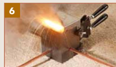
Once started, the reaction will take 3-4 seconds during which it is recommended to stand back the mould.
